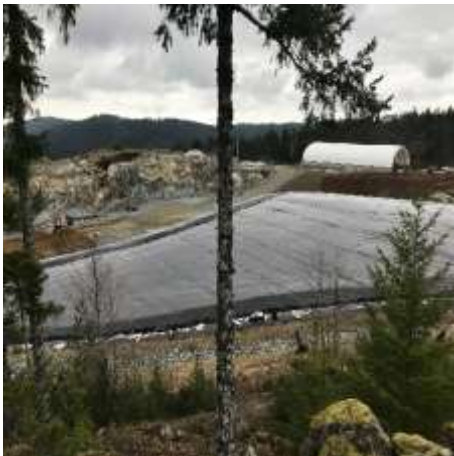
Site – Looking Northeast
