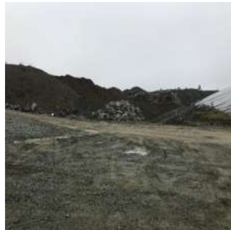
Soil Stockpiling – Looking South
