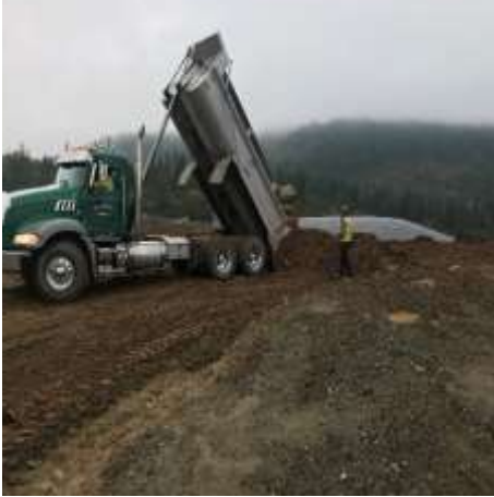
Site Stockpiling – Looking Southwest
