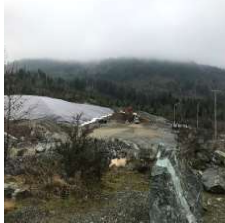
Site – Looking West
