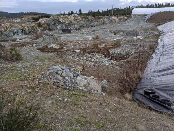
Site – Looking Northeast to Leachate/Leak Detection Facility
