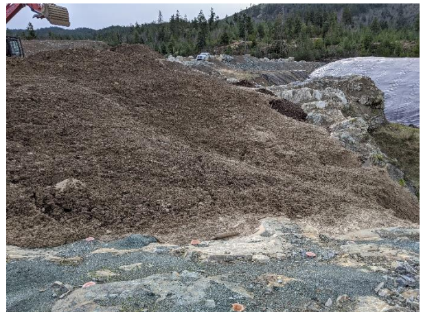
Soil Stockpiling – Looking southwest
