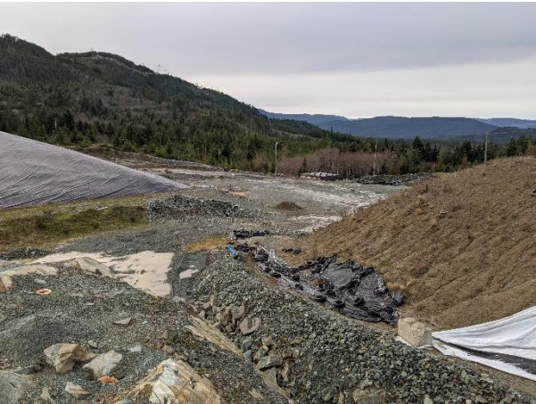
Site – Looking Northwest
