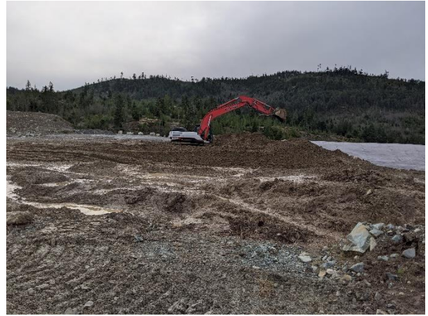
Soil Stockpiling – Looking West
