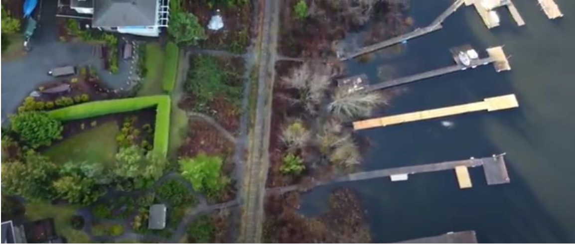
Aerial Photograph 6: Survey locations WP22 and WP23, north of Elford Road, Section 4/5 looking south (January 12, 2021)
